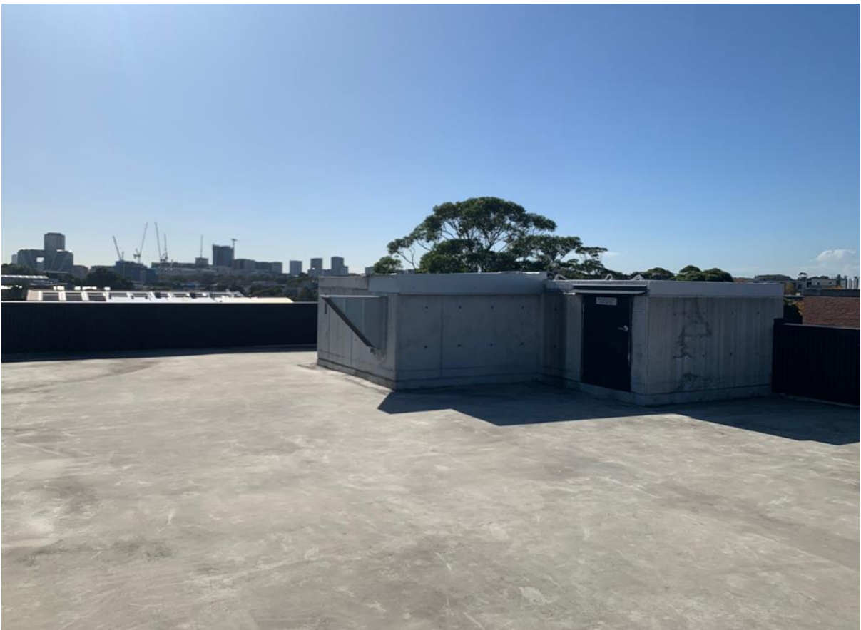
Figure 5: Existing rooftop showing fire stair access and mechanical ventilation
