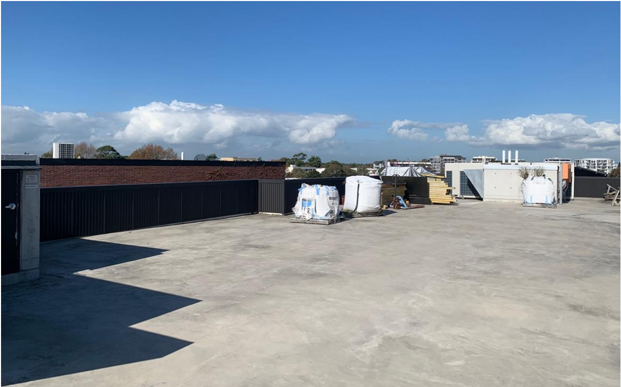
Figure 4: Existing rooftop of subject site
