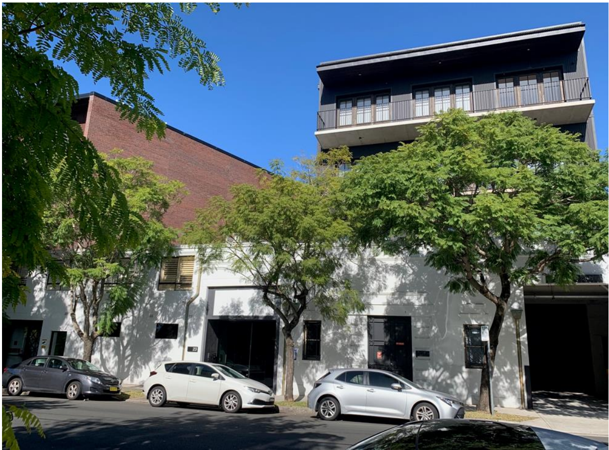
Figure 3: Doody Street frontage showing the blank wall of the neighbouring commercial building
